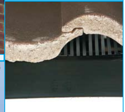
Eaves Protector with combed vent ▲
